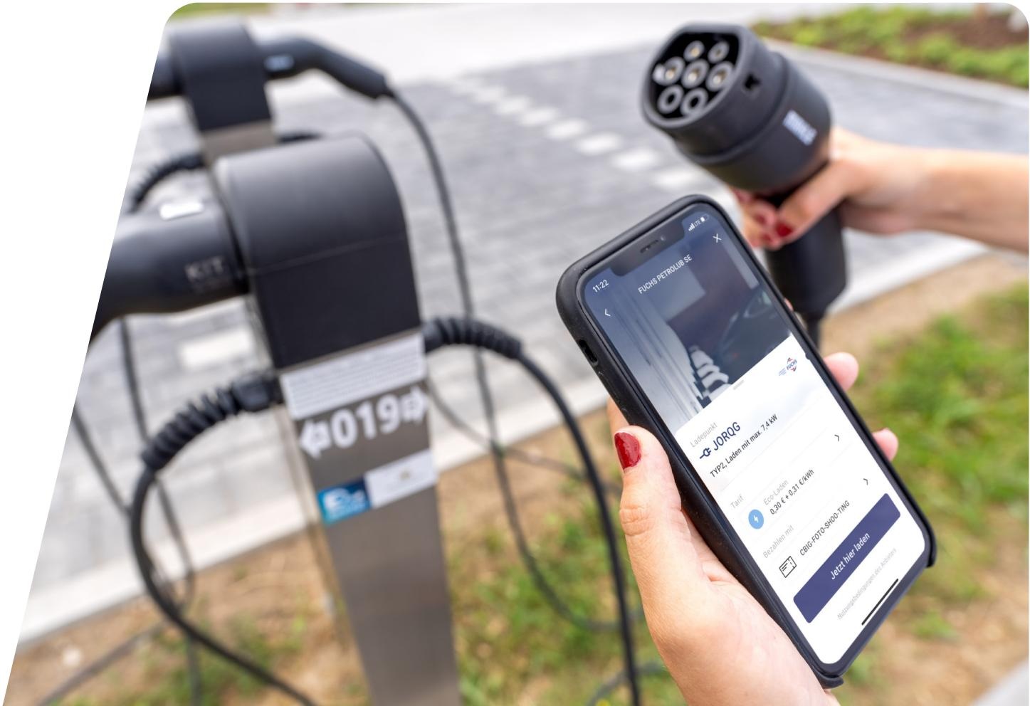
With the chargeBIG system, it is possible to construct many charging points despite a limited electric capacity in the grid infrastructure at the location. The existing grid connection is used optimally and intelligently. Expensive peak outputs are also avoided. By customer request, the load management communicates with other consumers or producers, such as a photovoltaic system in the grid. chargeBIG uses the electric vehicles as a controllable load.
